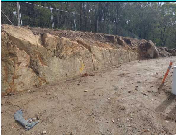
Photograph 5: Area of Excavation
