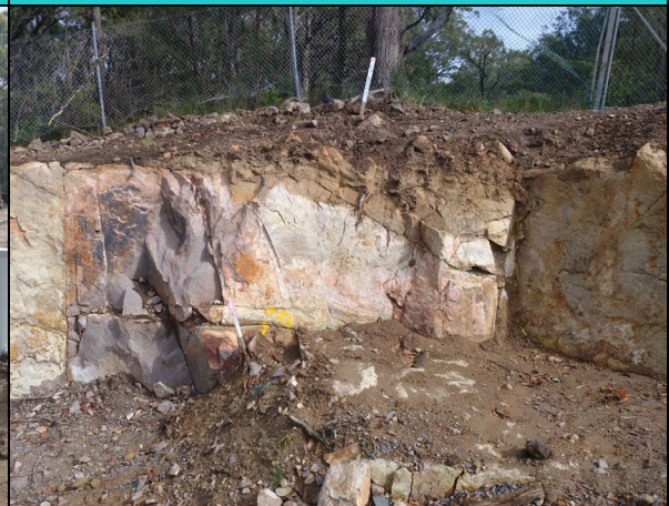
Photograph 6: Area of Excavation
